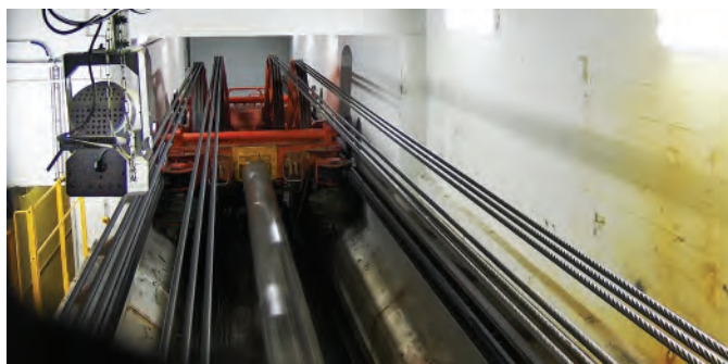
Fig. 5. Chriot pulling the cables in the subbasement. Credit: France Languérand.
